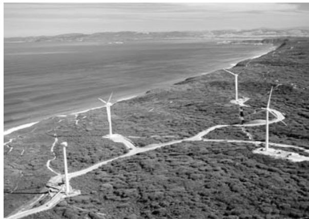
Albany wind farm, W.A.
